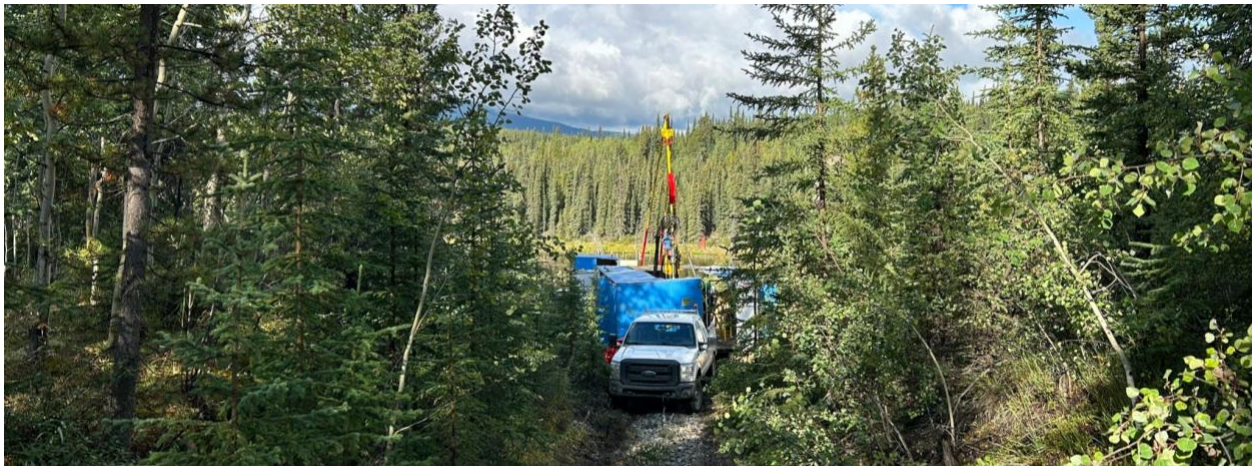
Drilling at Cowley Park – August 2024
